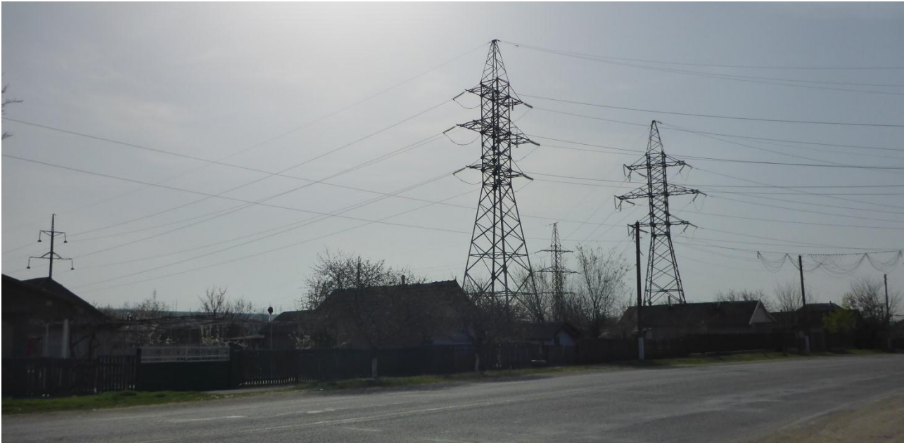
Figure 4.7.5 Houses build close to existing OHL
