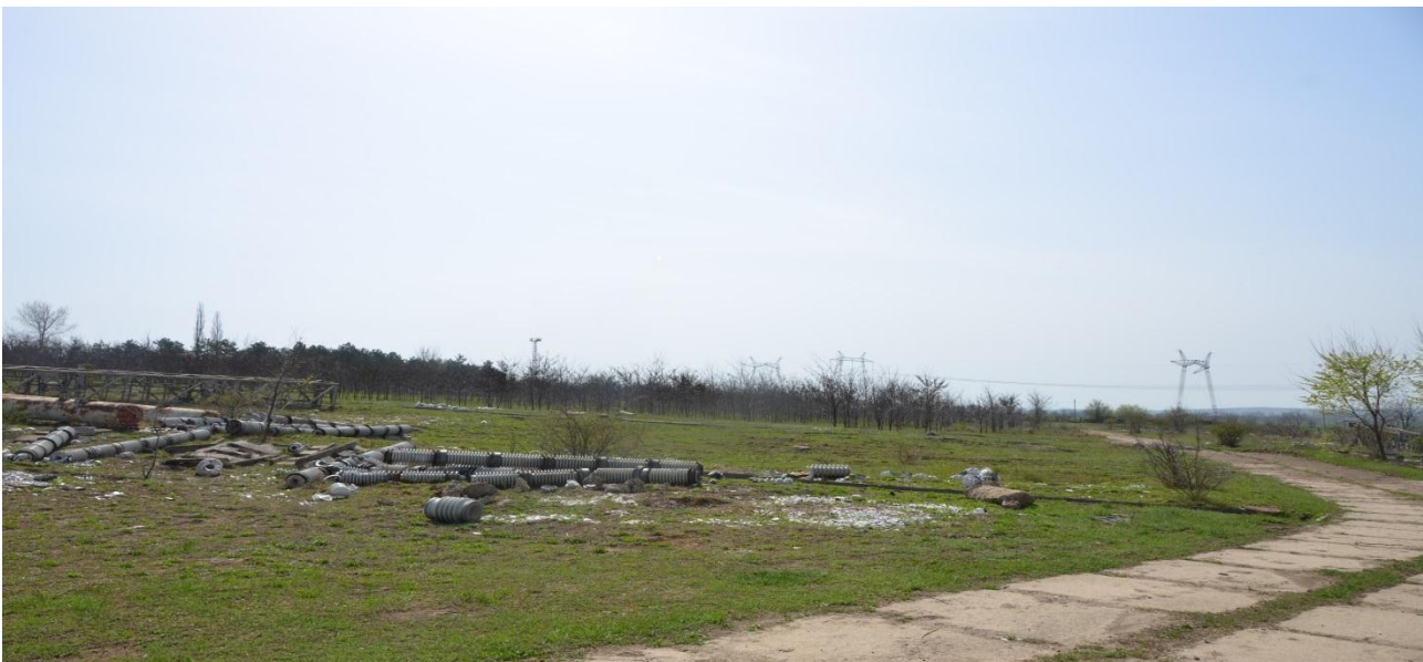
Figure 3.1.1.2 The demolish site considered for the new sub-station, also note the accacia tree nearby
